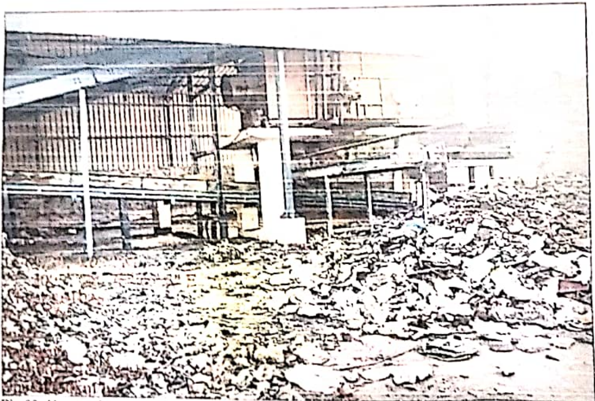
Fig 02: Heaps of segregated wastes from the ballistic separator were found at the site.
